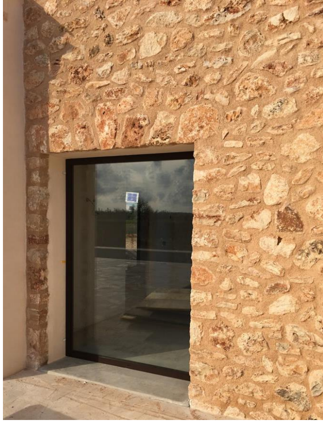
Stone massony walls
