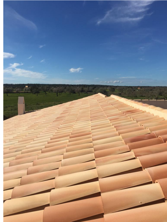
Ceramic roof tiles, concealed guttering and brick chimney
